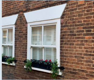
Sash window with lintel above
